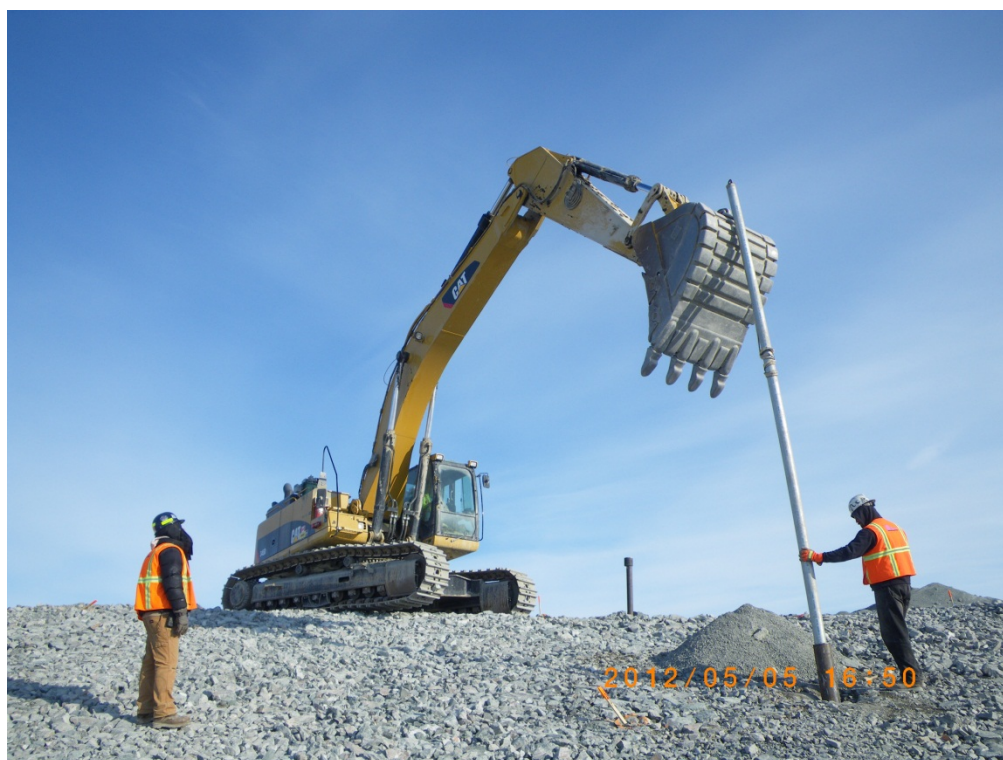
Photo 3: The Deep Settlement Pipe being lowered into the outer steel casing of ND-DSP-100.
