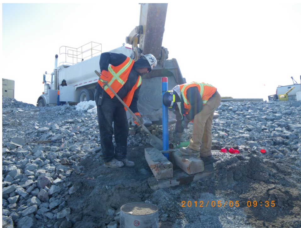
Photo 2: Installation of the last Inclinometer Casing into ND-IN-070-1.
